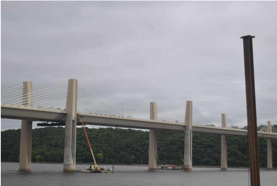
Crane barge used to hoist temporary access platforms (Kraemer previous project)
