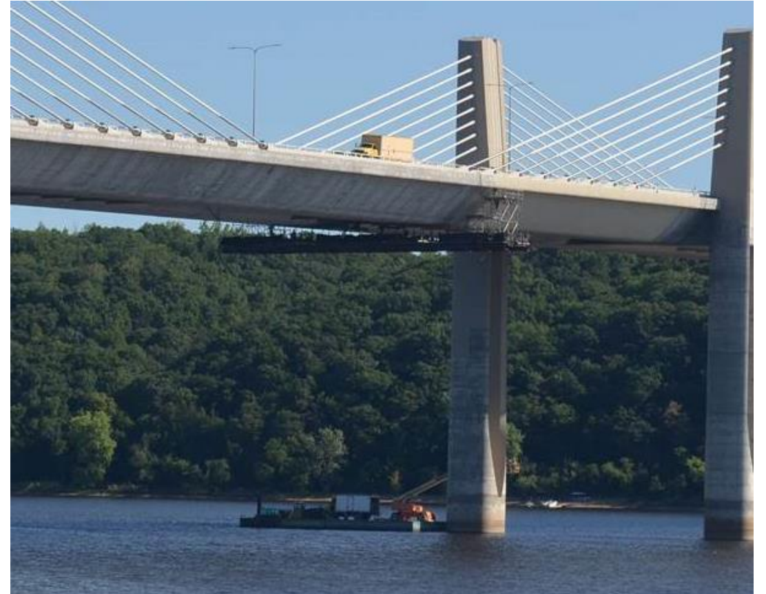
Temporary access platform (Kraemer previous project)
